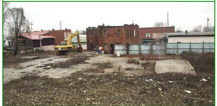
BEFORE: Demolition of the old scrap yard and Odd Fellows building
