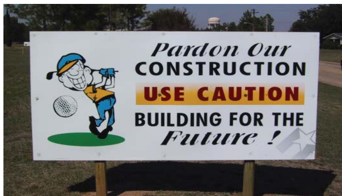
Sign at construction site
