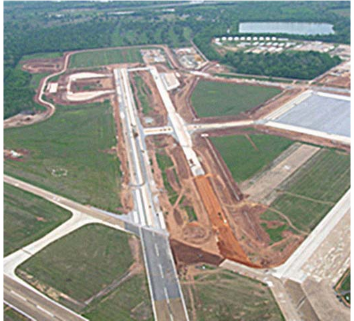
Aerial view of runways at England Air Force Base
