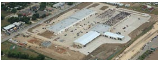
Aerial view of the 25-acre parcel/James Avenue Service Center under construction
