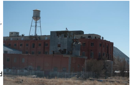
Former Sugar Beet Factory located in Eaton, CO
