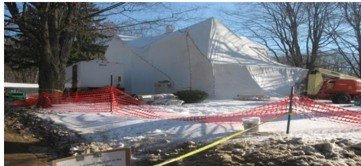
Decontaminating a residence in Danbury, Connecticut
