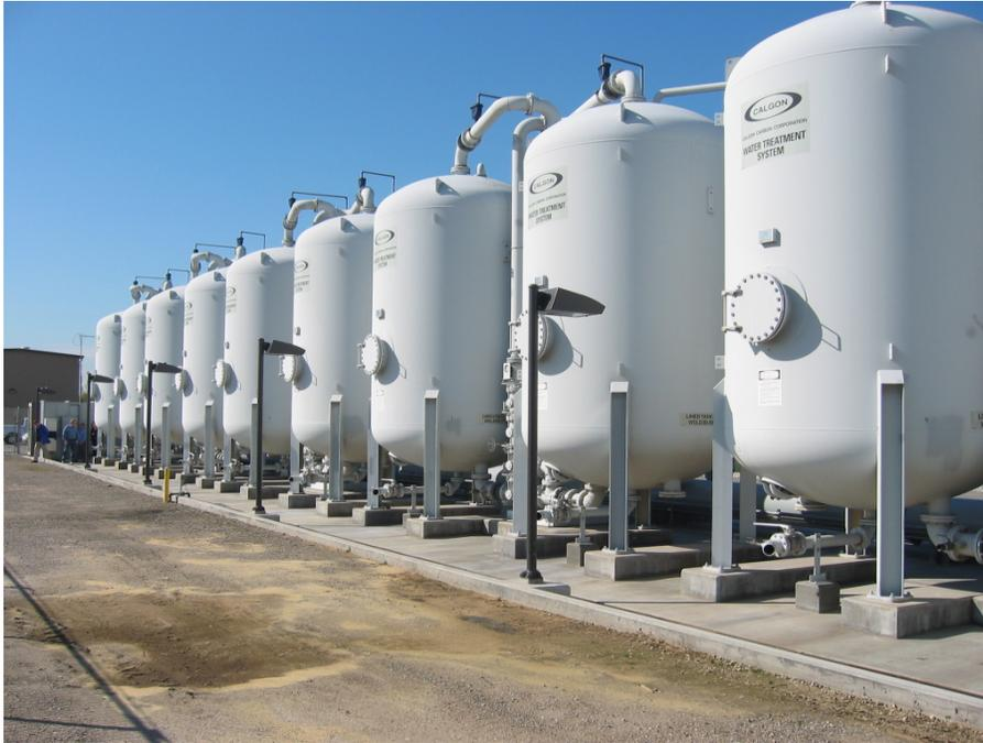
**Figure 3-5. Single Pass Ion Exchange System Installed at California Domestic Water Co.**
