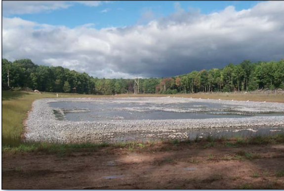
Figure 2. Vertical flow limestone treatment pond.
