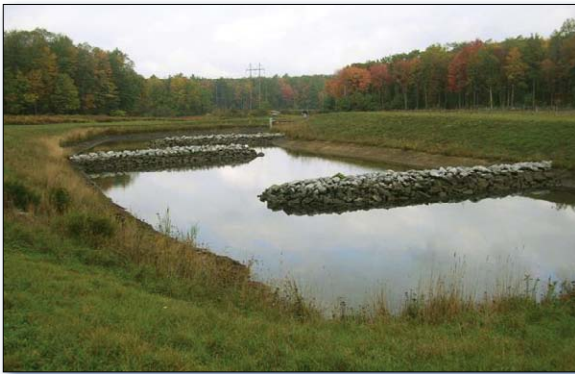
Figure 3. Settling pond with limestone baffles.
