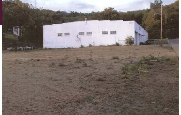
Above: Remediation in process.
