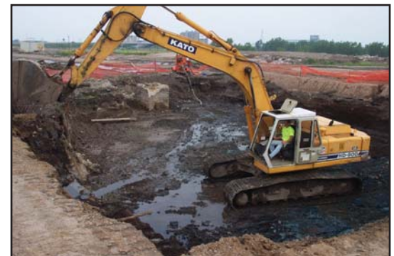
Petroleum cleanup in progress.
