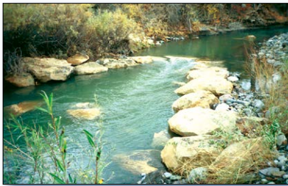
Figure 3. Project partners installed cross vanes and other stream channel stabilization BMPs.
