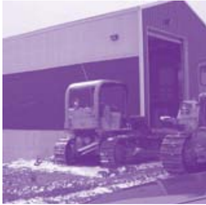
Turtle Mountain's new transfer station.
