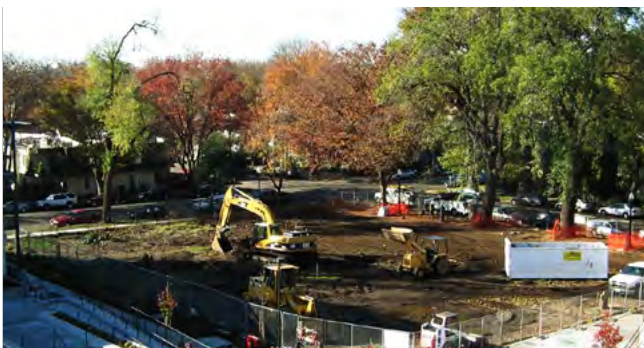
Construction underway at the Fremont Community Garden - Sacramento, CA
