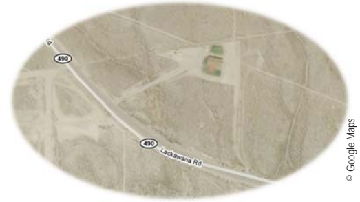
Aerial view of the Ely Landfill.
