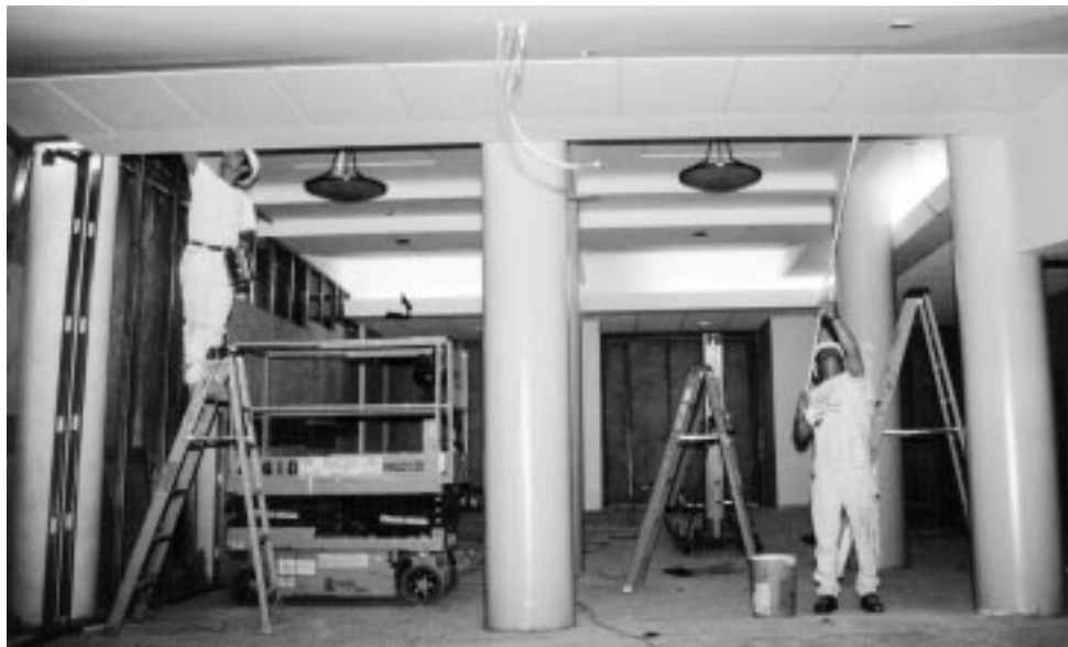
Paints used as part of the renovation were screened for environmental preferability.
