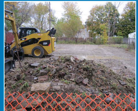
Large amount of demolition debris removed from soils at this site highlights the importance of planning ahead for solid waste removal and recycling.
