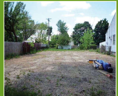
Site after demolition.
