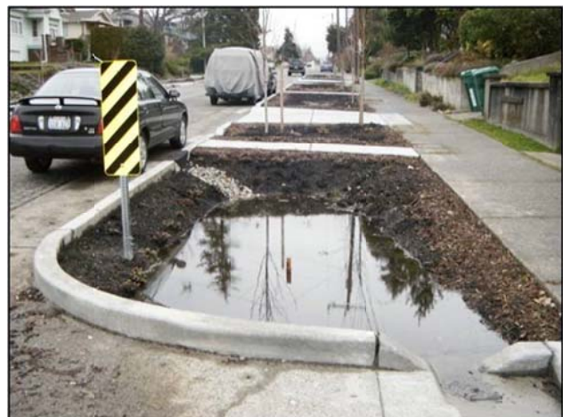
Figure C - Full Curb Shift Example
