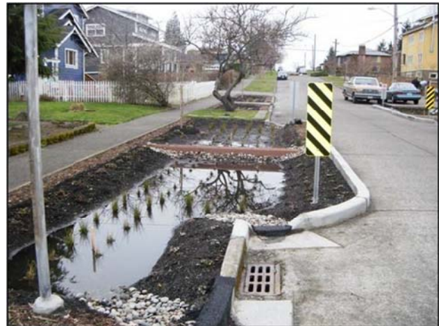
Figure B - Curb Extension Design Example
