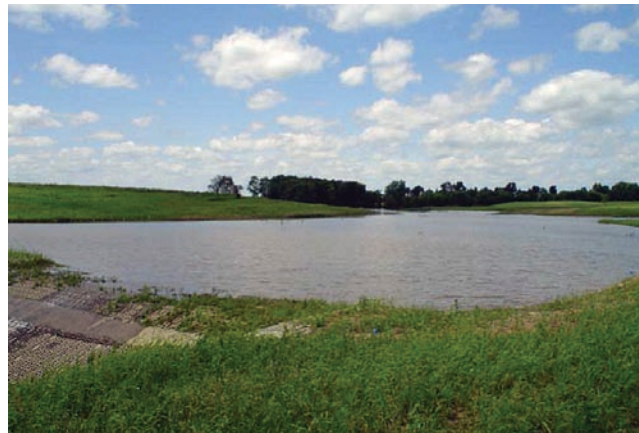
Figure 2. Stormwater wetland basin: post-construction.
