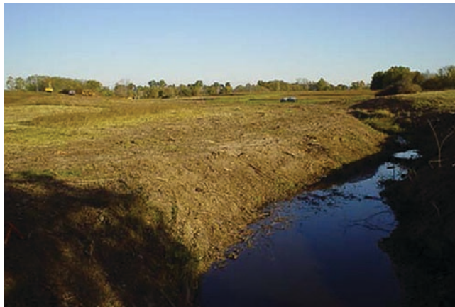
Figure 1. Stormwater wetland basin: pre-construction.
