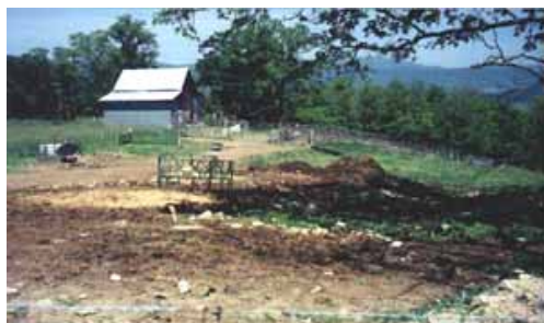
Example of a concentrated animal feeding area prior to BMP installation.
