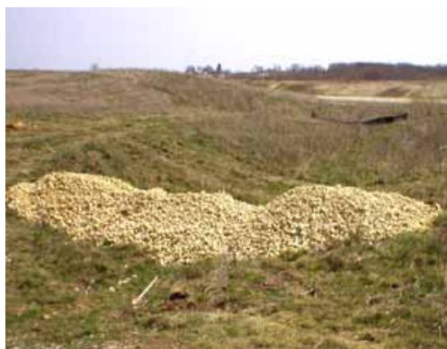
USRWA points to local developer Capitol Underground as a model for others to follow. The company installs and maintains silt fences as needed, grades the site in small phases, leaves grassed buffers, and places piles of crushed stone in runoff ditches (called “stone weepers”) to slow water and prevent sediment from leaving the site.
