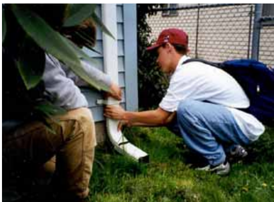
Volunteers help disconnect a downspout.
