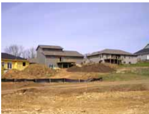
USRWA points to local developer Capitol Underground as a model for others to follow. The company installs and maintains silt fences as needed, grades the site in small phases, leaves grassed buffers, and places piles of crushed stone in runoff ditches (called “stone weepers”) to slow water and prevent sediment from leaving the site.
