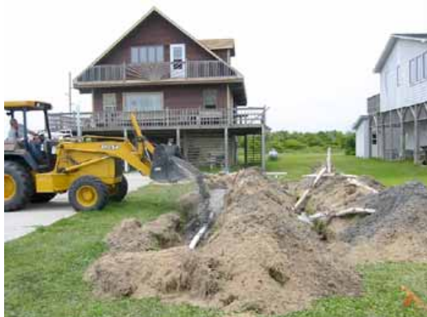
Contractor performing drainfield repair for a loan recipient.
