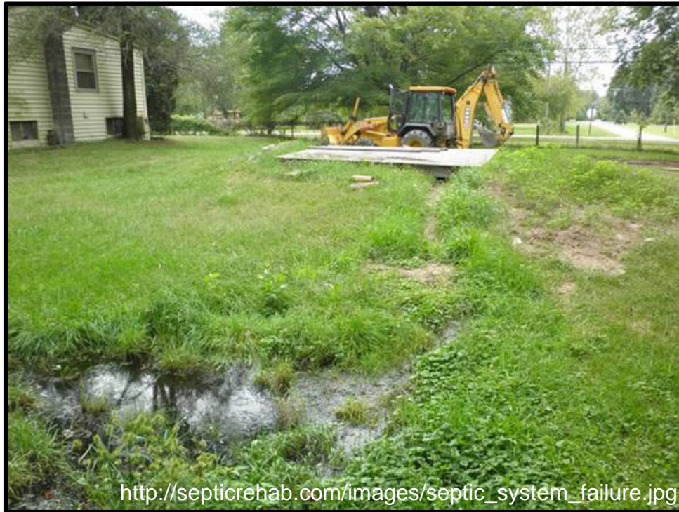
Failing septic system
