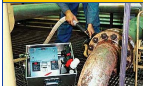
Exhibit 2: Leak Measurement Using a High Volume Sampler
