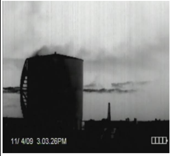
Exhibit 4 View of tank emissions using the infrared camera.
