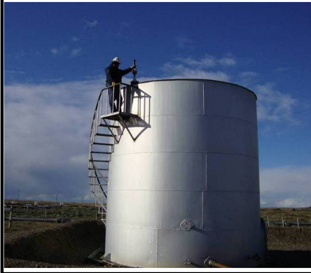
Exhibit 3 A measurement expert uses a turbine meter to quantify tank emission rates.
