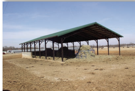
Areas for cattle feeding and waste storage were constructed to reduce the amount of bacteria and nutrients entering the stream.
